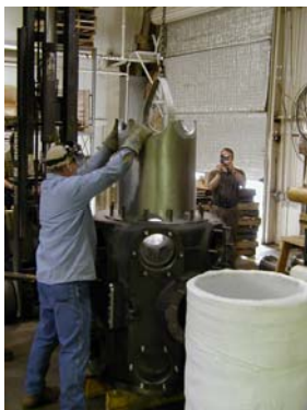
Installing a new 20.5 in. (520.7 mm) bore, shrink fit liner into the bore of the new cylinder body. Prior to insertion, the liner was “soaked” in liquid N 2 to provide radial clearance for installation.
